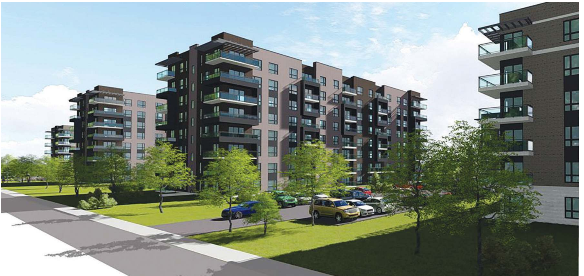
Le Seville West aims to immerse residents in green spaces, create community, and provide the convenience of city living. Note: photo is a rendering. SUPPLIED
